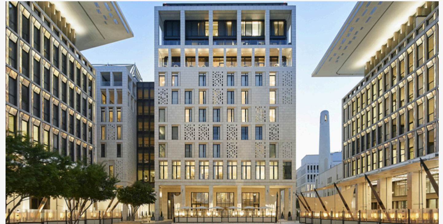
Msheireb Downtown, Doha, Qatar
